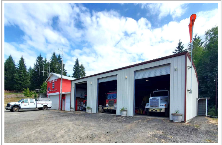
Station 1 after volunteers scrubbed it down, hauled away debris, and added planters.
