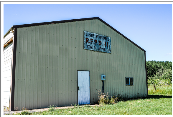
Station 3 had been in disrepair for several years, with rats nesting inside in the apparatus and the insulation, and safety hazards throughout.
